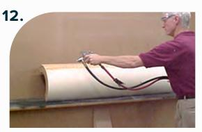
Apply contact adhesive to column face.
