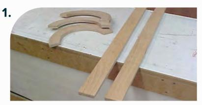
Cut horizontal ribs as needed. Horizontal ribs should be placed every 15" to 18". Attach vertical rails to the length of the column.
