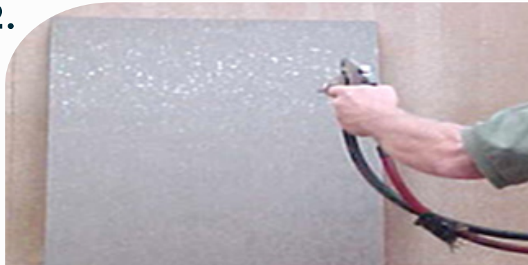
Apply adhesive to back of veneer.
