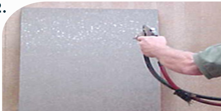
Apply adhesive to back of laminate.
