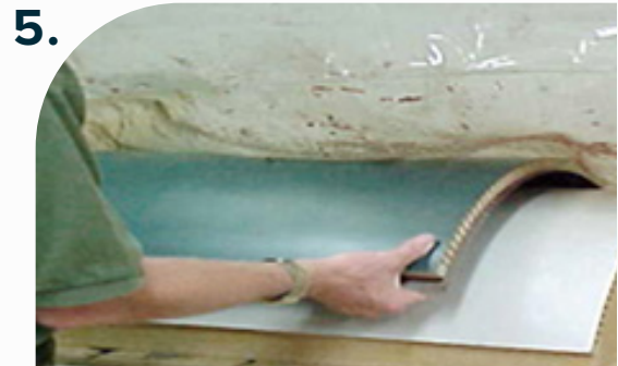
5. Place HPL face down on form. Then, place Soflex with glued rib side down onto HPL.
