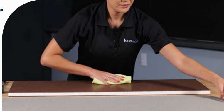
Clean the surfaces by removing all dust and debris.
