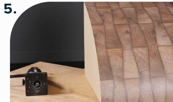
Use a router to remove excess material from edges.
