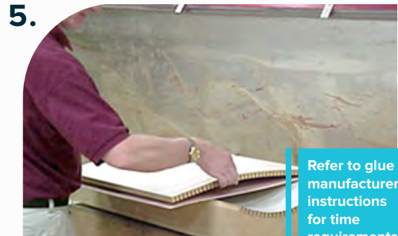
Position Timberflex and back panel together over form.
