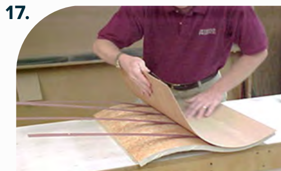
Position decorative material on door.
