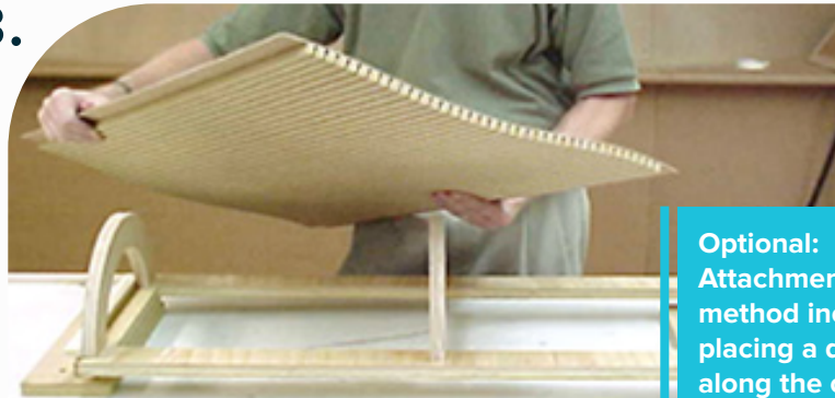
Use a pre-sized, pre-laminated flat piece of Kerfkore. Lay across the ribs using glue. Kerfs should run vertical with the length of the column.
