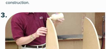
To attach Flexboard, the framework should consist of horizontal ribs.
