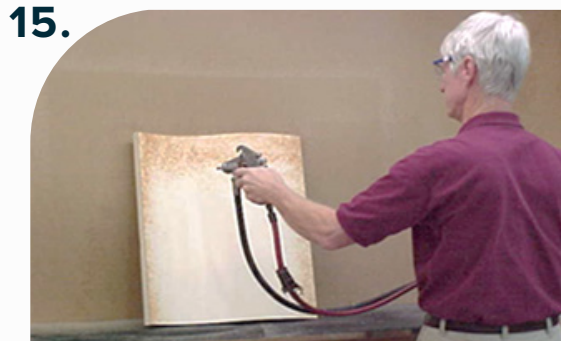
Apply contact adhesive to door face.
