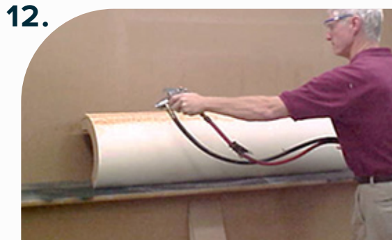
12. Apply contact adhesive to column face.
