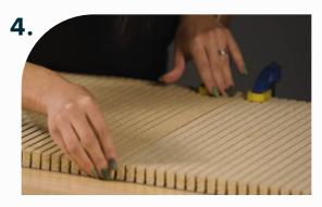
Place seam rib over seam, maintain a 1/8" gap on either side, press and hold.
